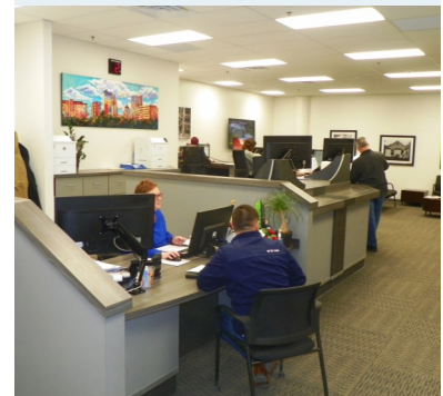
Remodeling work in the Allen County Building Department offices was finished in the early part of 2019. The completed project included a remake of the front counter and reception area. The work was done by the County Buildings and Grounds Maintenance Department.
