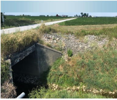
Antwerp Road Bridge (photo courtesy A&Z Engineering)
