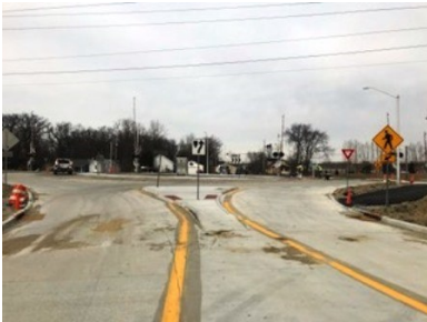
New Bass-Hadley Road Roundabout
